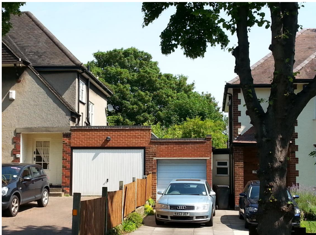
Photograph 5 from Hillcrest Ave between Nos. 17 & 19 (closer view)
